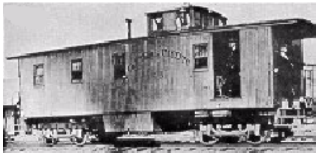
Central Pacific No. 45, built in August 1872 with wood frame trucks, could seat 22.
