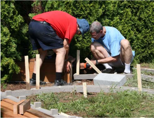
The removal of the arborvitae allowed Richard and Rex to install the tunnel through the hedge.
