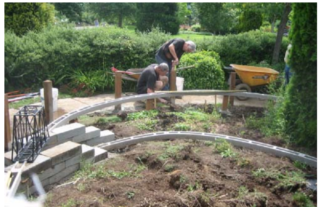
Work in progress (photo by Penny Walker)
