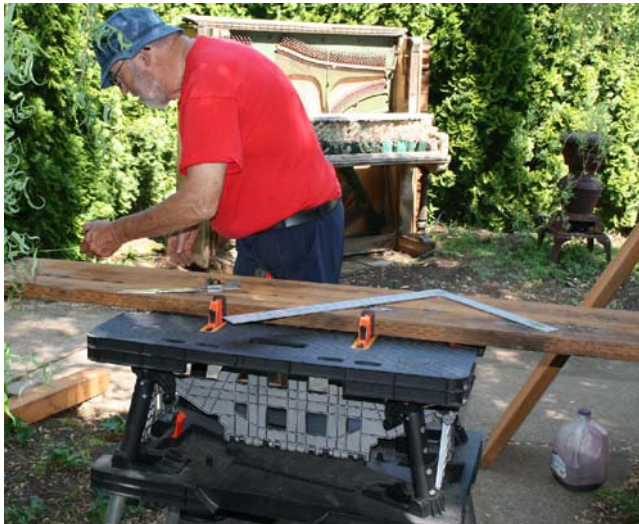
Richard Walker cuts wood for the tunnel
