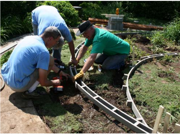
It took three sets of hands to put the second side on the sub-roadbed.
