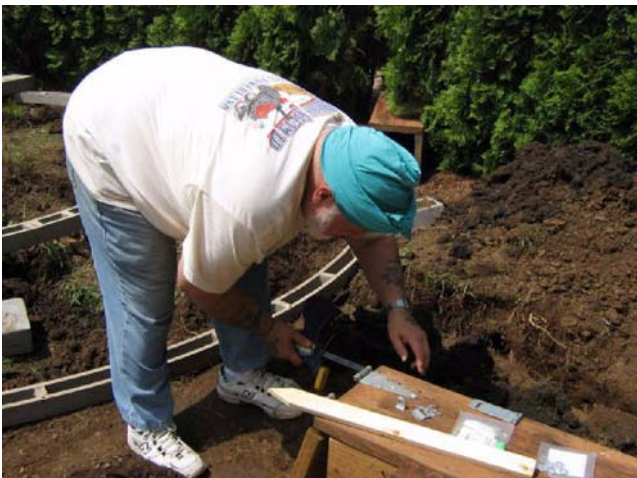
Jim Greer builds the train storage shed.
