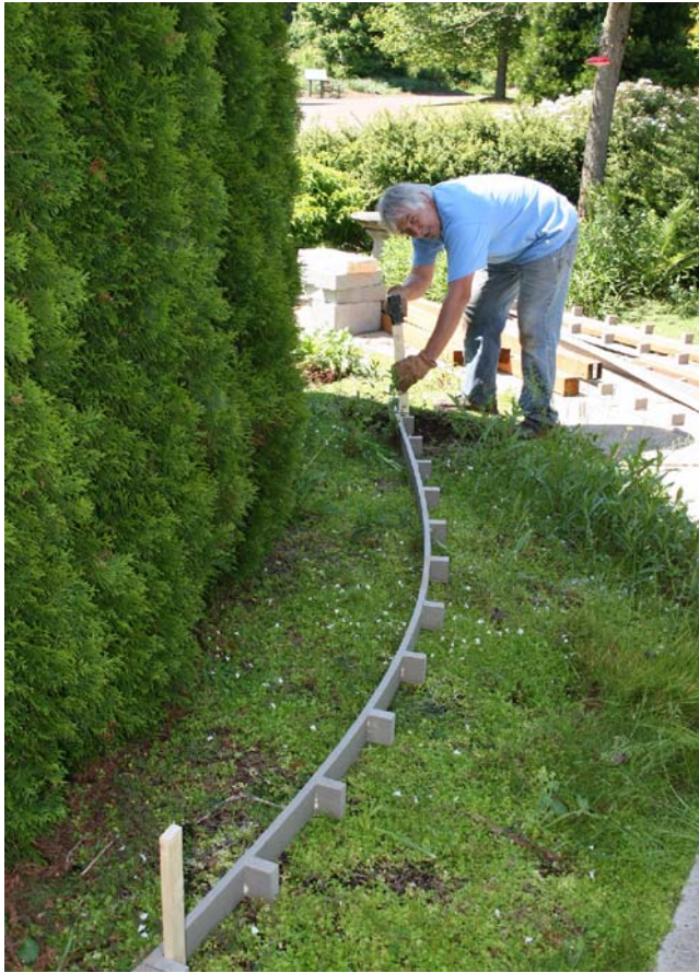
Installing the sub-roadbed
