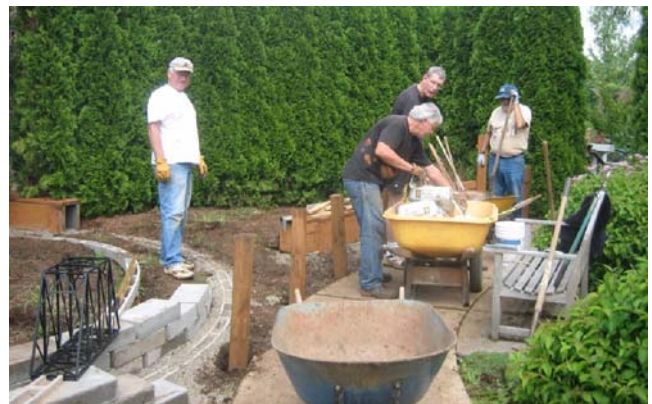
Work in progress (photo by Penny Walker)
