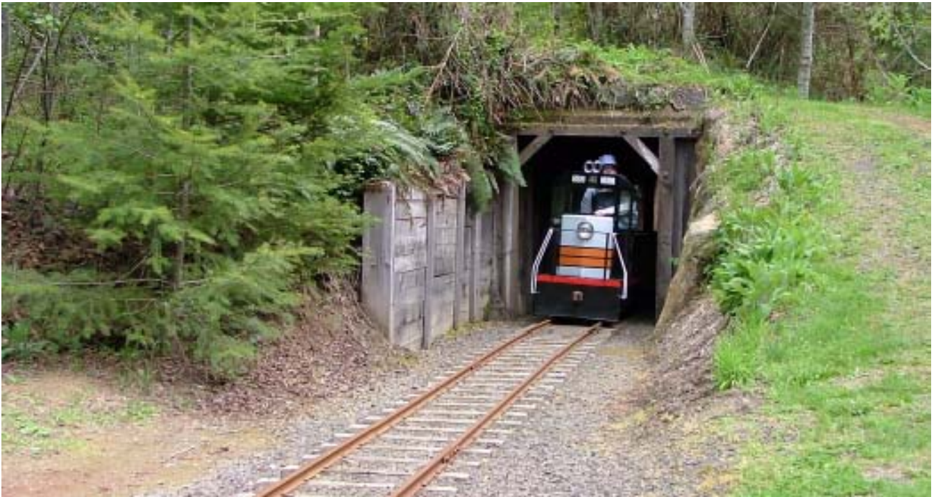
The tracks follows Deadwood Creek and passes through a tunnel.
