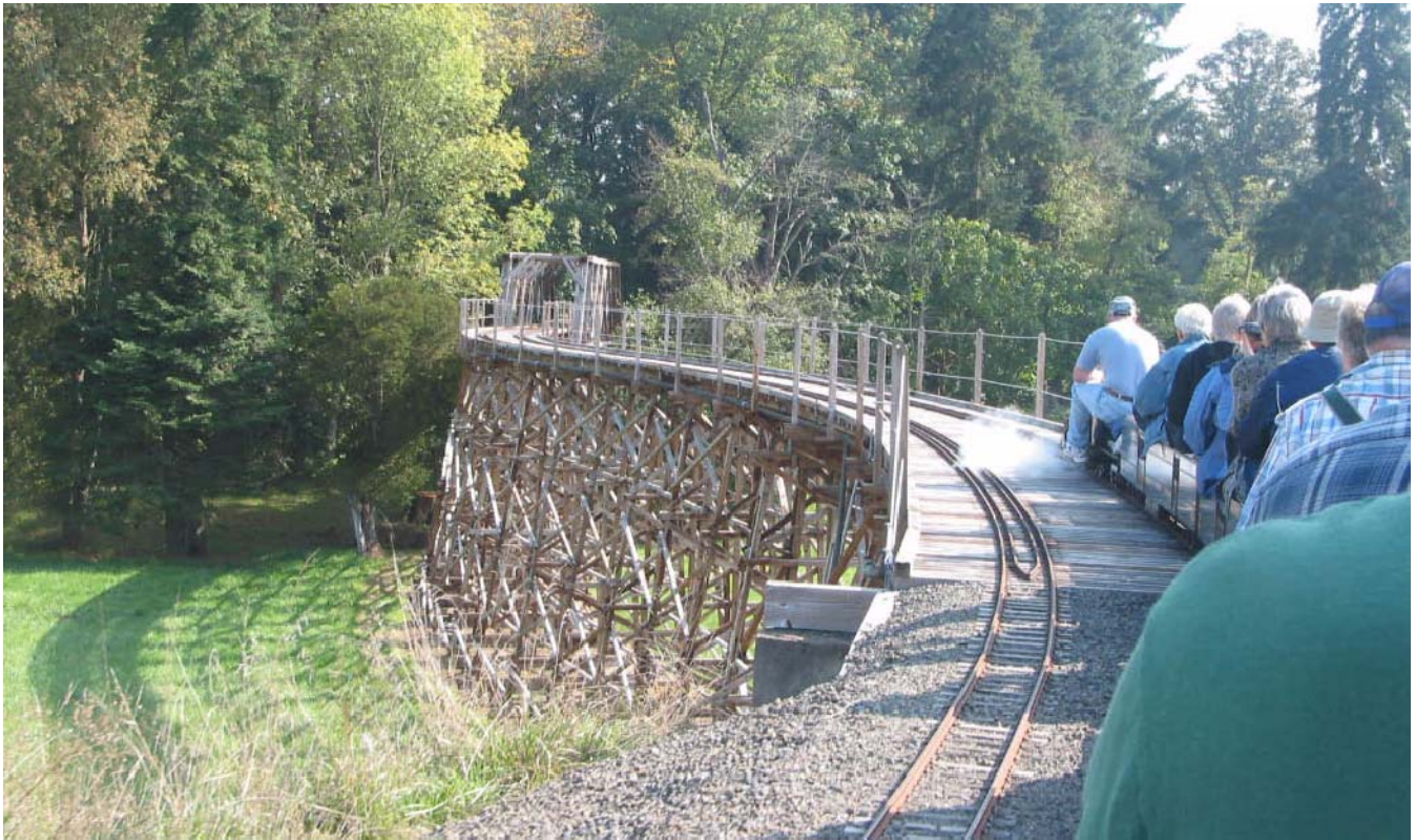
A full load of passengers cross the 400 foot trestle and through the Howe truss bridge. The timber used in the trestle and bridge are dimensioned to the scale of the railroad.
