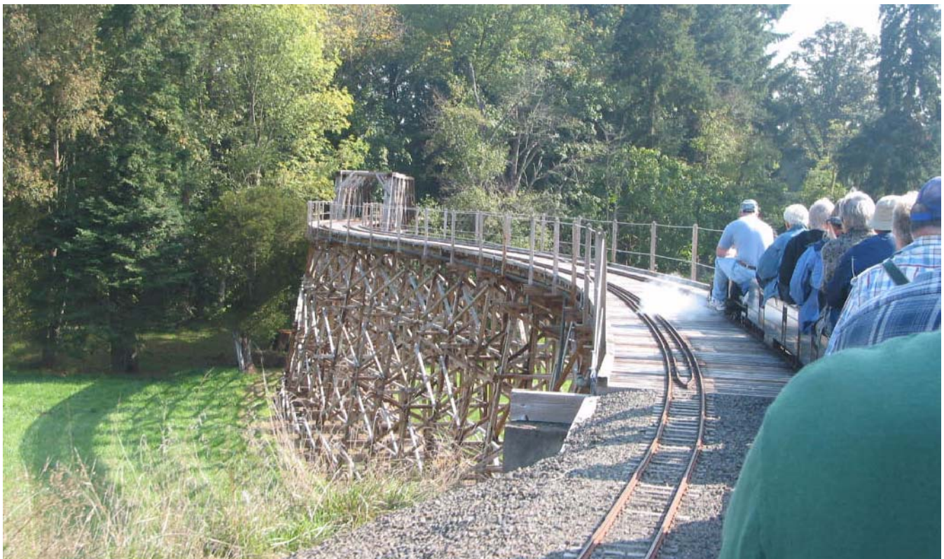
The 4-4-2 "Atlantic" takes a full load of passengers across the 400 foot trestle and through the Howe truss bridge.
